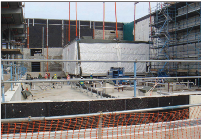
Modules set on foundations.
