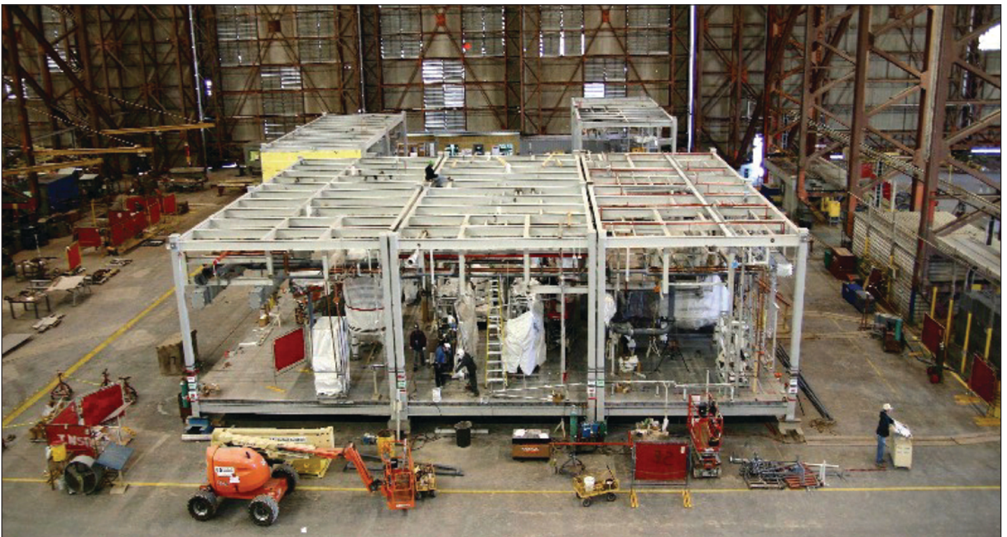
Modules staged in final layout.
