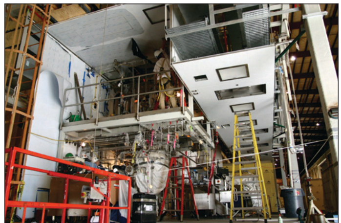
Module fabrication shop.
